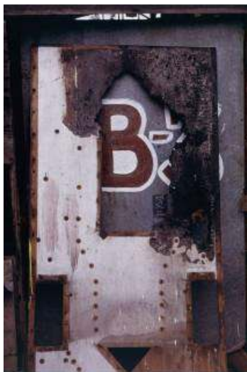
Figure 31: Side wall of a re-circulating batch dryer that caught fire
