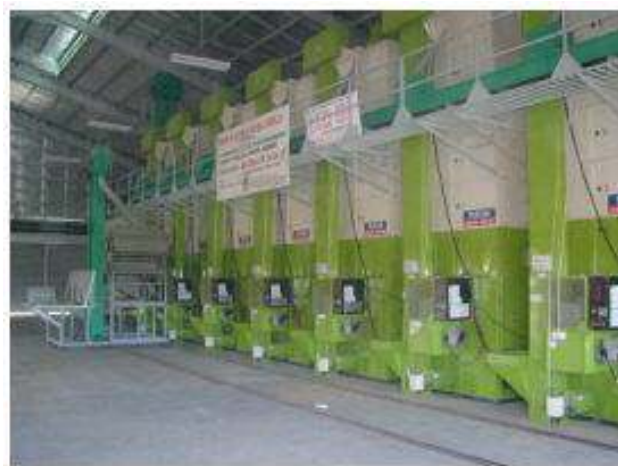
Figure 18: A row of re-circulating batch dryers in a Philippine rice mill
